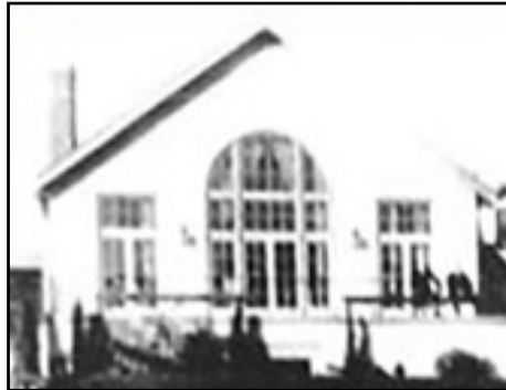
The south wall of the church in 1925 this at length and factored in the input of a structural engineer.
