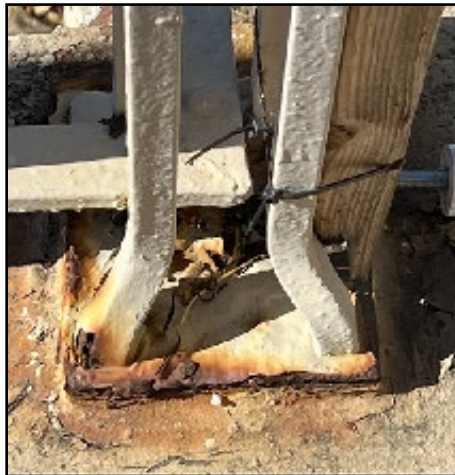
Examples of railing failures.
